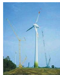
Figure 4. The ENERCON E112, a 114 metre diameter wind Turbine, hub height 124 metre, with a direct drive variable speed generator rated at 4.5 MW.
