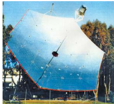
Figure 3. The 400 m 2 Parabolic Solar Collector at the Australian National University, Canberra
